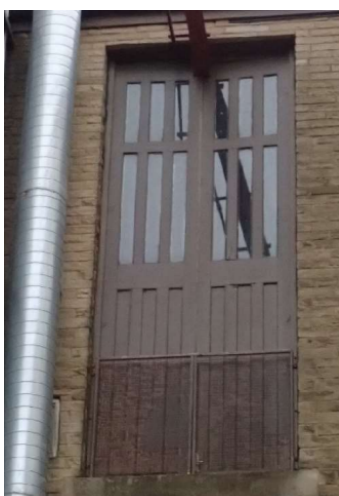
Existing First Floor Doors
